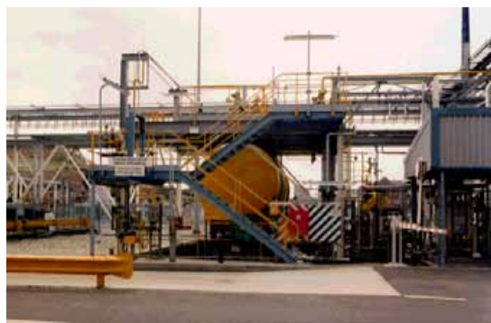
A well designed unloading area
