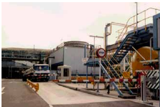
Tanker waiting to enter unloading area
