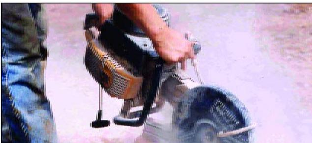
**Figure 2** Sawing – dry
